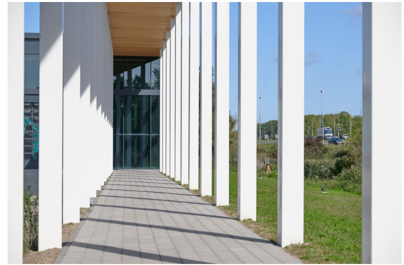
Kobelco connection between buildings
