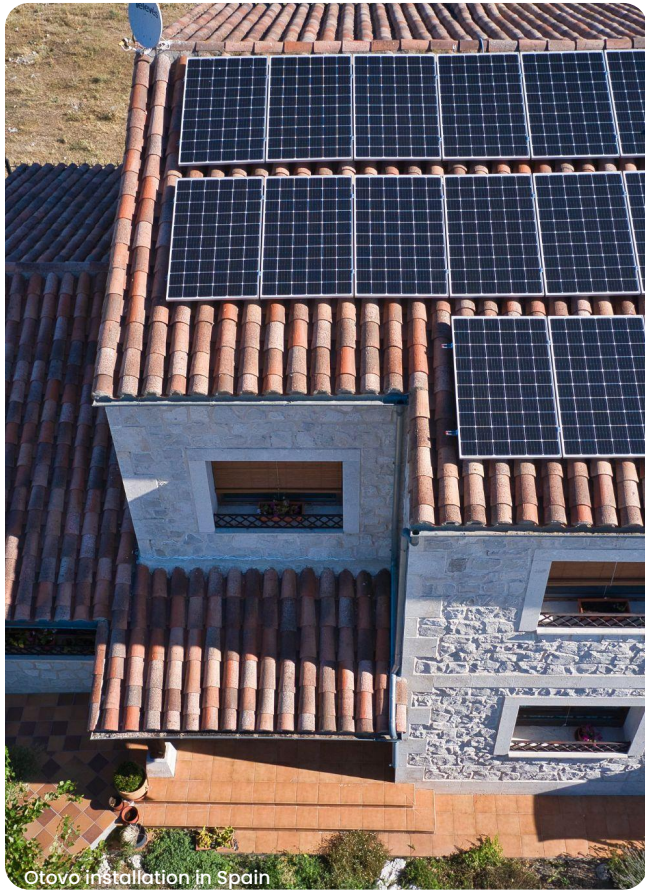
Otovo installation in Spain
