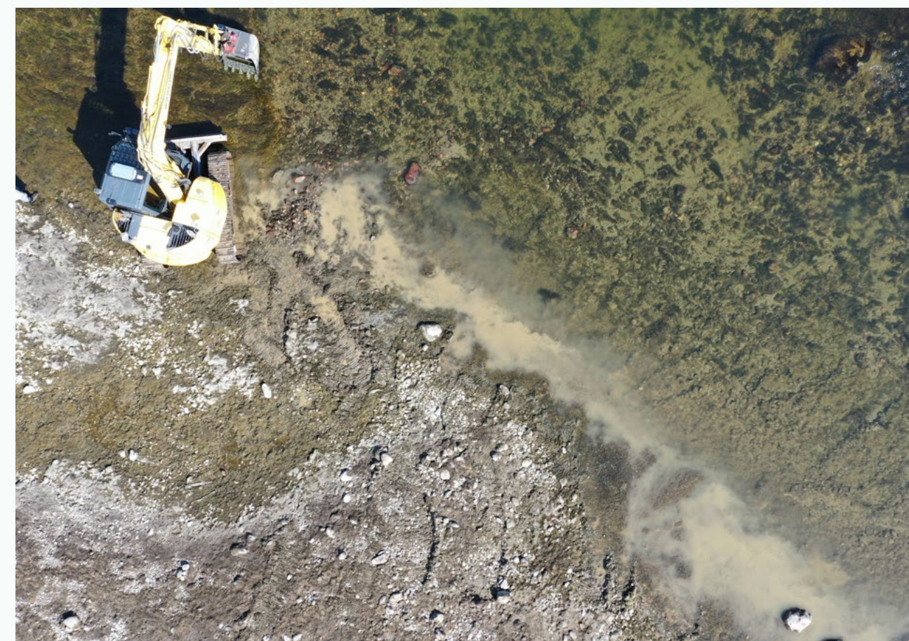
Repair of the river bottom in Vorma.
