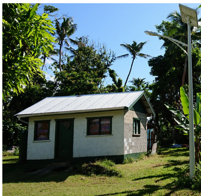
Concrete block house with CGI roof sheeting in Tongatapu. CC- Leo Gaggl
