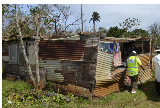
Reuse of metal roofing sheets for walls. House in 'Eua. © Bill Flinn- Care
