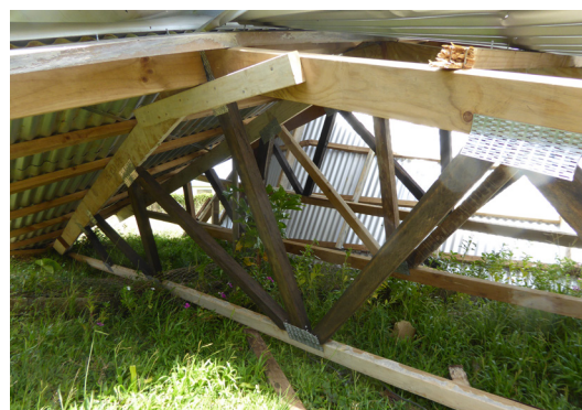
This roof, not having been firmly connected to the walls, was lifted off, due to the strong, vertical pressure (suction) of the wind. © Bill Flinn- Care
