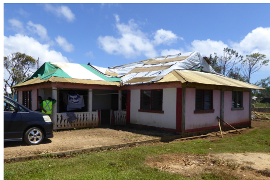
Plastic sheets on top of a damaged roof after cyclone Gita in 'Eua. © Bill Flinn- Care
