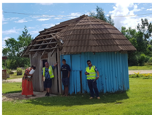
This damaged fale afa house can be repaired by reinstalling the lost roofing sheets/tiles. © IFRC
