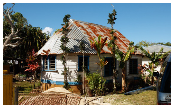
Fale afa with the oval shape of a fale built with concrete, timber and CGI sheet roof. © Douce Cahute maison-monde.com
