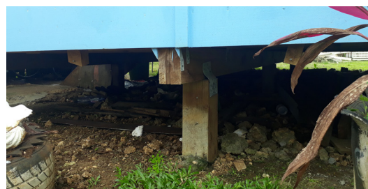
Tying down is important to resist cyclones. Fale afa house in Tongatapu. © Shelter Cluster Tonga
