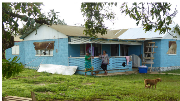
House with a veranda built with concrete blocks and CGI sheets roof in 'Eua. © Bill Flinn- Care
