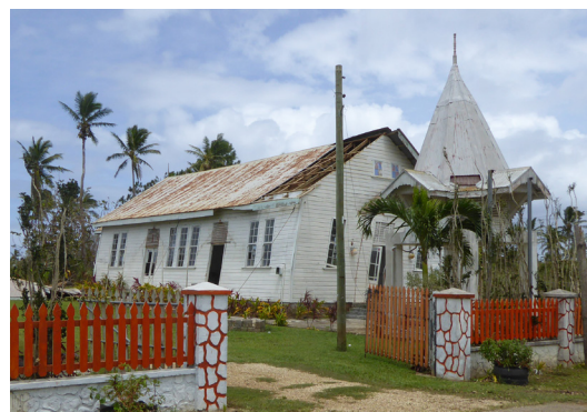
Church in Tongatapu affected by lateral wind probably because of a lack of bracing. © Bill Flinn- Care
