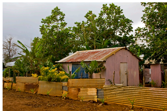
House with corrugated (CGI) roof sheeting and wall cladding in Vava'u. CC- clr_flickr
