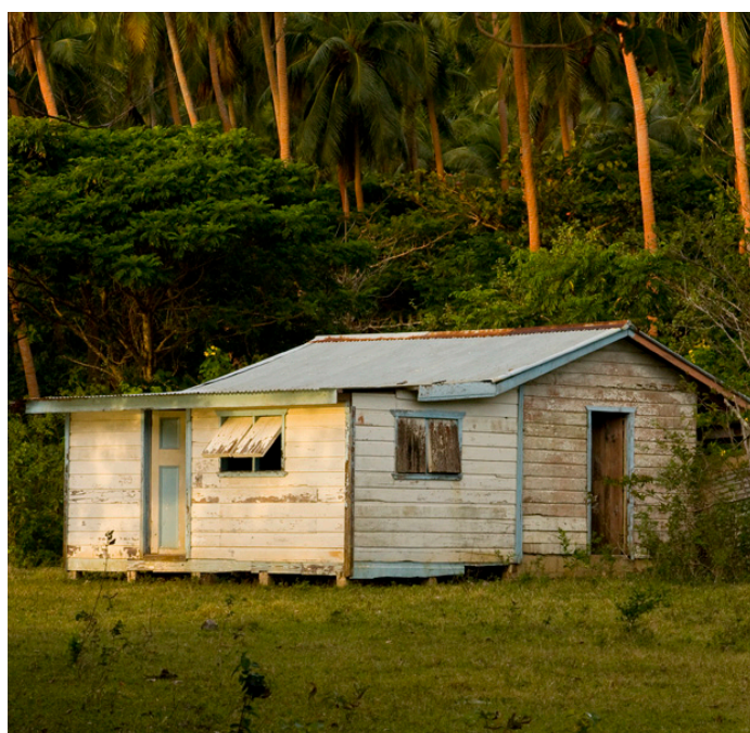
House with timber framed and clad walls and CGI roof sheeting on Kapa Island. Vava'u group.CC- clr_flickr
