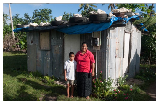
Heavy objects are often placed on the roofs to reduce the risk of wrenching of the CGI roofing sheets. © Caritas
