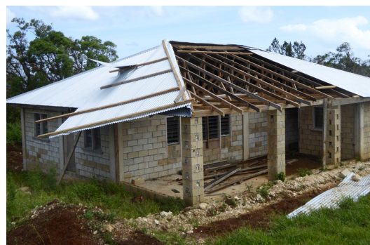
A veranda without ceiling and sharing the roof with the whole house may cause the entire roof to lift off in case of strong winds. House in 'Eua. © Bill Flinn- Care
