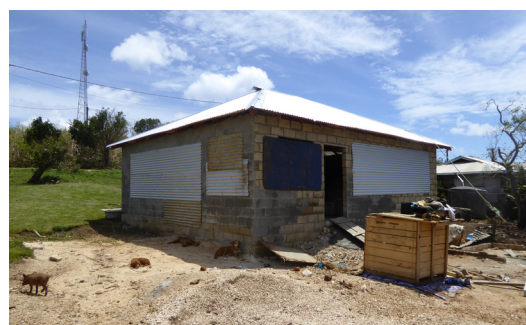
Hipped roof with better resistance to strong winds. Square shape with better resistance to earthquakes. House in 'Eua. © Bill Flinn- Care
