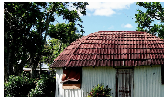
The roof tiles delay the sun's heat transfer through the metal. CC- Leo Gaggl
