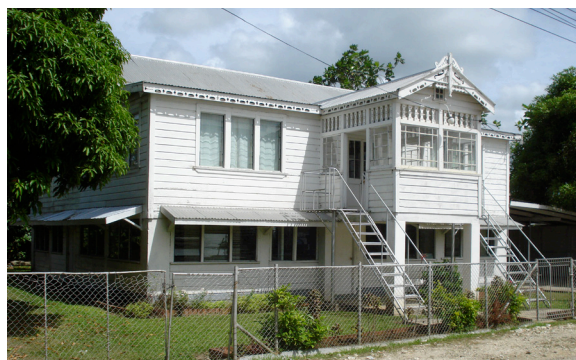
Two-storey building built with concrete structure and timber walls. CC Jen Crothers-
