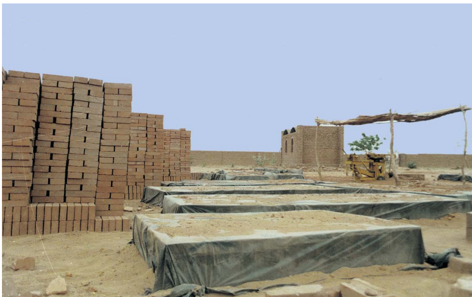
Figure 4.1 - Brick curing
