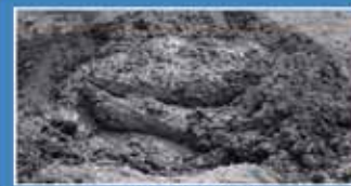
MIXING IN WATER. Mix in water gradually and use up within 90 minutes of mixing with water
