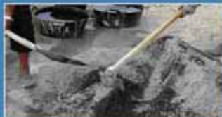
MIXING SAND GRAVEL AND CEMENT Not completely mixed until the color is uniform
