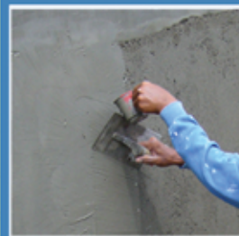
Finish the wall with cement-water slurry
