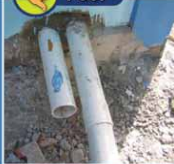
INADEQUATE DRAINAGE Graywater drains into foundation
