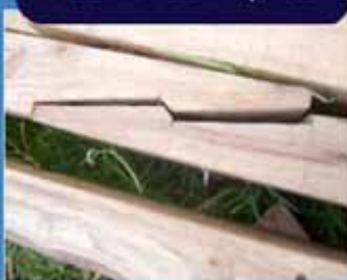
Beam-Beam Splice
