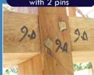
Fasten each joint with 2 pins
