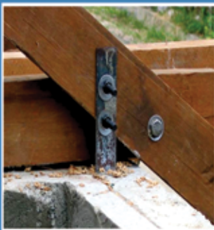
U-shaped plate in the ring beam
