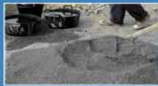
MIXING SAND GRAVEL AND CEMENT Thoroughly mixed dry ingredients.
