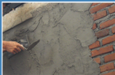
Use pressure to apply the plaster to the wall; do not just throw the plaster against the wall
