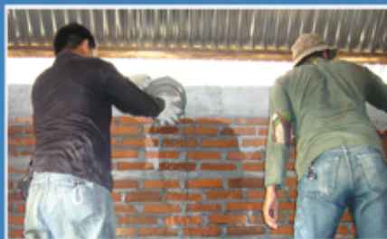
Wet the wall before applying plaster
