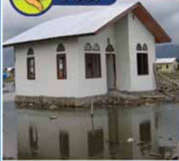
INADEQUATE DRAINAGE Poor grading and site selection
