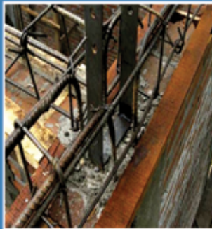
U-shaped plate in the ring beam
