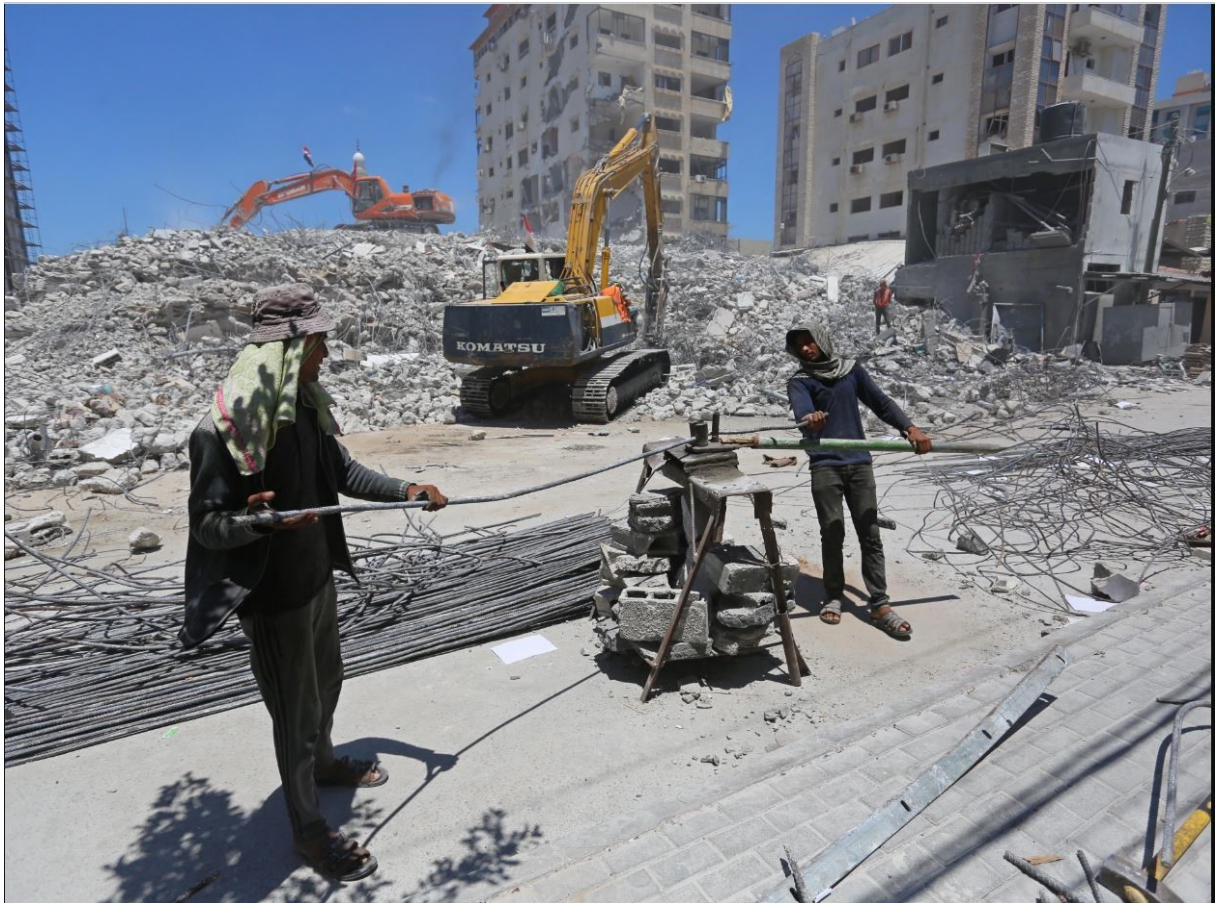
Gazan workers adjust rebar from damaged housing units for reuse in casting secondary concrete items.
