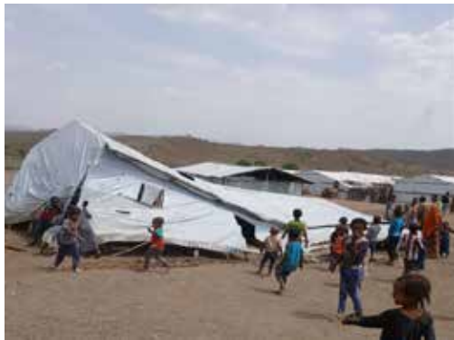
Photo credit Samaritan's Purse - Damage on emergency shelter due to heavy rain and wind storm, Jara, Amhara.
