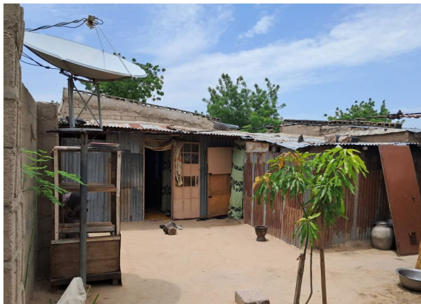
Recycled boards walls, Malakyariri, Borno state - © UniMaid
