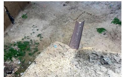
Proper maintenance of the evacuation of an earthen roof, Gashua, Yobe State - © UniMaid
