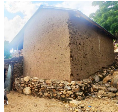
Foundations with stone, Gwoza, Borno state - © UniMaid
