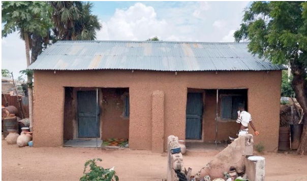
Earth walls and mono-pitch zinc roof, Buniyadi, Yobe State © UniMaid
