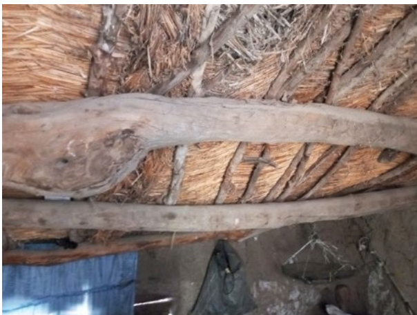
Earth roof with timber structure (a), Ngala, Borno State - © UniMaid
