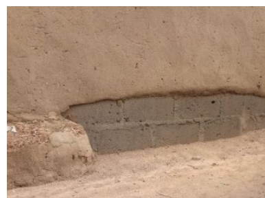
Sandcrete blocks in foundation of an earth wall, Fufore, Adamawa state - © UniMaid
