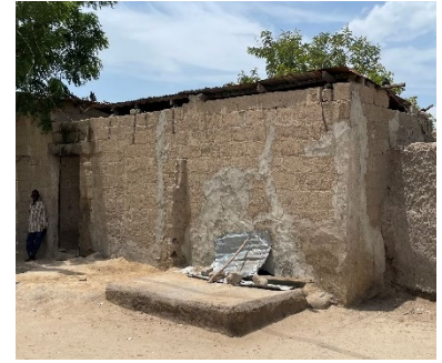
Cracks on sandcrete walls due to proximity to septic tank, Rabiri Community, Dikwa, Borno State - © UniMaid
