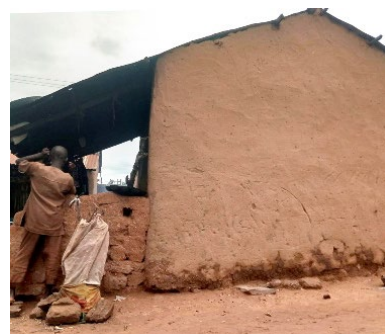
Damaged wall because it lacks of foundations, Wuroahi Community, Fufore, Adamawa State - © UniMaid
