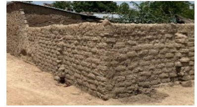
Mud bricks wall, Dikwa, Borno state © UniMaid
