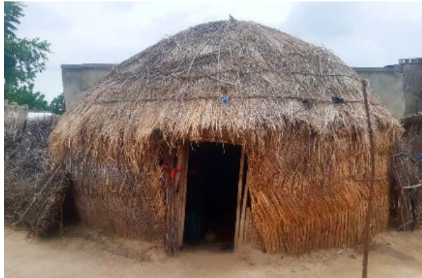
Thatch walls and roof, in Dikwa, Borno State – © UniMaid
