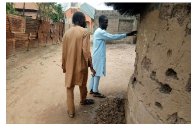
Earth walls requiring re-plastering maintenance, which is more difficult if the plaster is stabilised, Opalo village, Lamurde, Adamawa State - © UniMaid
