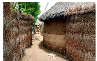
Sandcrete blocks foundation under earthen walls avoids rising humidity, Opalo, Lamurde, Adamawa State - © UniMaid
