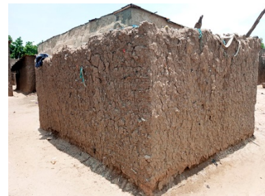
Erosion of the lowest part of the wall. Potiskum, Yobe State - © UniMaid
