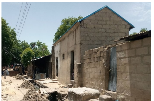
Cement walls, gable zinc roof, Bulabulin, Borno state - © UniMaid
