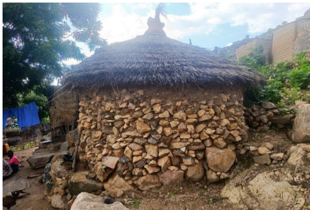
Stones and earth with thatch roof in Gwoza, Borno State - © UniMaid
