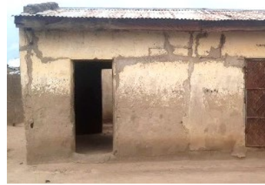
Cracks on sandcrete walls due to the lack of a ringbeam, Bulabulin community, Dikwa, Borno State - © UniMaid
