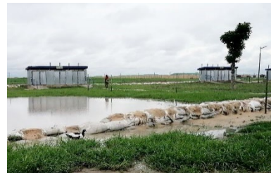
Sandbagging, Dikwa, Borno State - © UniMaid
