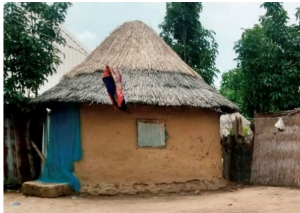
Mud-bricks and thatch roof in Opalo, Lamurde, Adamawa State © UniMaid
