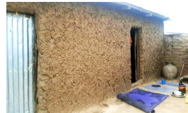
Earth plaster with fingerprints, Bulabulin Community, Dikwa, Borno State - © UniMaid
