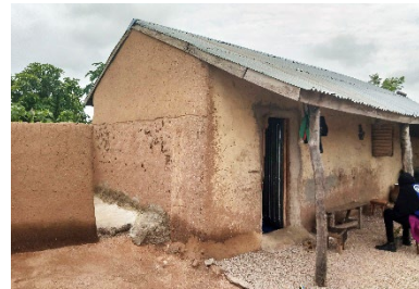
Cement slab next to earthen wall causes damage to wall base, Gombi, Adamawa State - © UniMaid
