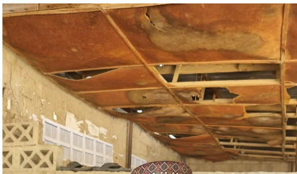
Plywood needing repair, very often because the roof covering is leaking on it, Malakyariri, Borno state - © UniMaid
