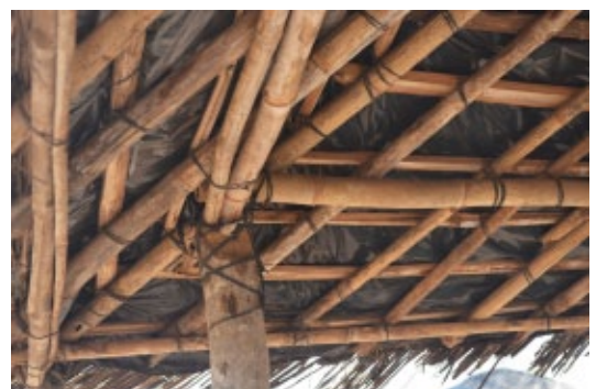
Plastic sheet membrane in a roof in Chipile, Mangochi. © Jon Twingi
