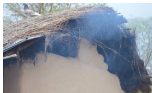
Kitchens always present openings to let the smoke out. Smoke has very bad impacts on people's health, but at the same time it treats thatch against insect attacks: Thatched roofs let the smoke out more easily as they are porous (William, Rumphu). © Jon Twingi
