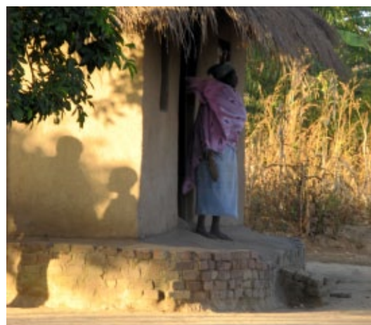
Some families protect the ends of the raised earthen mound with fired bricks or stones. House in Mtetera. CC- Firesika.
