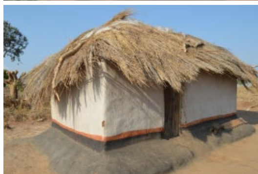
Low-rise houses with round and compact forms and symmetric and scarce openings and light roofs are good to resist seismic forces. Round house in Kachipeso, Dowa (top). Square house in Muwanga, Chitipa (bottom). © Jon Twingi
