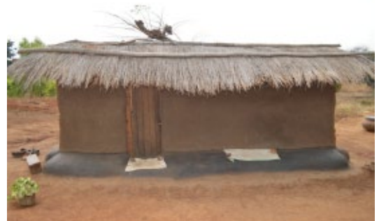
House built on a raised platform with wattle and daub walls and thatched gable roof. Mkalawa, Rumphi. © Jon Twingi
