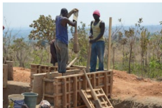
Many constructions in Malawi are built using local, renewable materials with little impact in the environment when they are well managed. This image shows the construction of a rammed earth house in Nisanje, Lilongwe. © Jon Twingi
