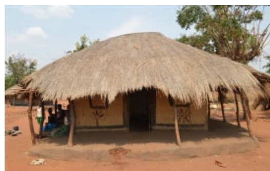
Verandas and large roof overhangs between the interior earth wall and the exterior avoid the risk that changes in humidity associated with rain will swell the soil under the walls. House in Simwaka, Nkhosakota.
