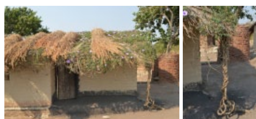
In some villages, the roof is used as a support for climbing plants. The risk of wrenching as well as partial or total uplift is reduced as the plants fasten together the roof components and attach the roof to the ground through the roots. House in Nsangu, Salima. © Jon Twingi
