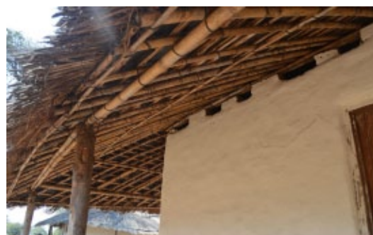
House in Dzibusile, Ntcheu. This house has a contact surface between the wall and the roof structure which is minimised using only some bricks to sustain the framework. This permits ventilation, but also allows for a better visual detection of termites paths and thus a better control of their attacks. © Jon Twingi
