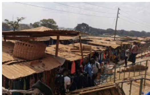
The use of CGI sheets without false ceilings and without ventilation in the gables causes thermal and acoustic discomfort. Market in Lilongwe. © Roderick Vd.
