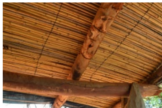
Reed is used as bottom layer in many roofs. Roof in Chome, Rumphi. © Jon Twingi.
