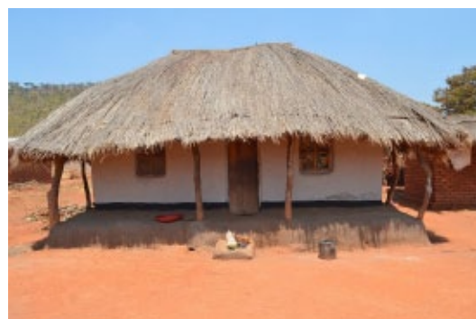
House built on a raised platform with a four sides veranda and a thatched hip roof and with its façades protected by a plastering and painted. Gama, Mchinji. © Jon Twingi .
