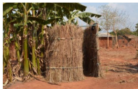
Latrines and showers are usually built using vegetal materials such as grass, timber, bamboo or reed.
