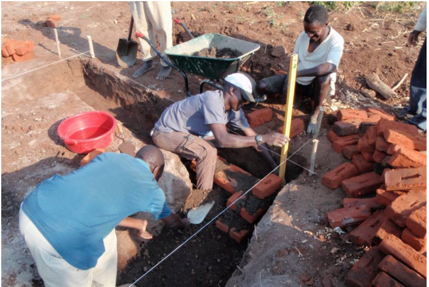
Construction of a foundation. CC- Gregory S.
