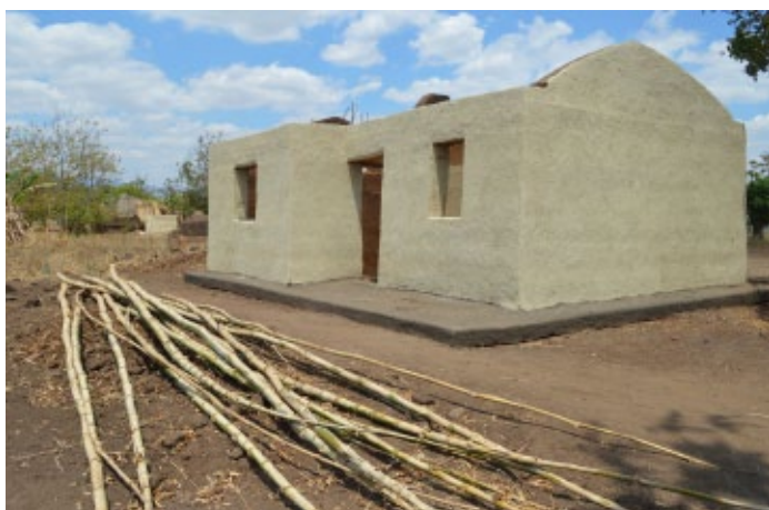
Rammed earth house under construction. © Jon Twingi
