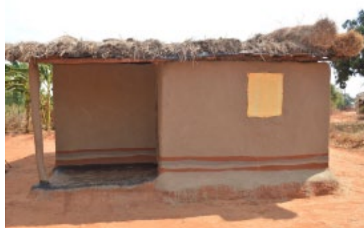
Thatched roofs are repaired when necessary. This house in Chome (Rumphi) presents thatch bundles which can be easily replaced when they get rotten. © Jon Twingi
