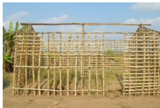
Light structures are good solutions in the event of an earthquake as even if they fall they are less likely to cause damages. Structure of a wattle and daub house in Mwaluwimba, Karonga. © Jon Twingi
