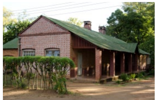
British colonialism also introduced in Malawi the use of fired red bricks, regular and paced windows and doors, concrete or burnt bricks lintels and roofs covered with corrugated iron sheets. Mission in building in Blantyre. CC- Carmichael C.
