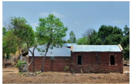
Corrugated galvanised steel or iron sheets are the most common metal roofing system in Malawi. Houses in Makala. CC- Hansueli Krapf
