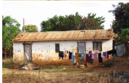
These two houses would be semi-permanent according to different authors as they are built with a mix of materials. The one on top has burnt bricks and thatched roof (Kachopatsonga, Nkhosakota Bay - © Jon Twingi). The other one has adobe brick walls and metallic roof (Lilongwe - © Urbanopolista)
