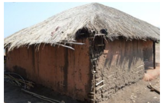
Maintenance of roofs is crucial to block water from penetrating the walls and to make them stay stable. House in Mwamwiyo, Karonga. © Jon Twingi
