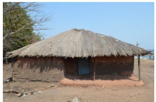
House with veranda built on a raised platform with wattle and daub walls and thatched hip roof. Mwamwiyo, Karonga. © Jon Twingi
