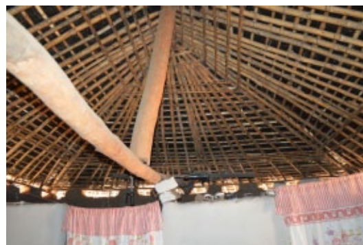
Bamboo is more and more used, for example in roof frameworks. Hipped roof in Dzipusile, Ntcheu. © Jon Twingi.
