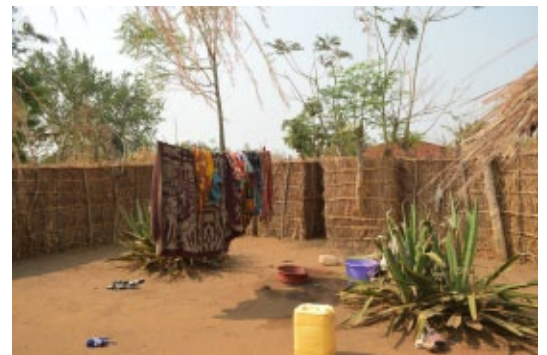
Bamboo, grass or reed fences are sometimes built to reduce the speed of wind and to delimitate plots. House in Lifidzi, Salima. © Jon Twingi
