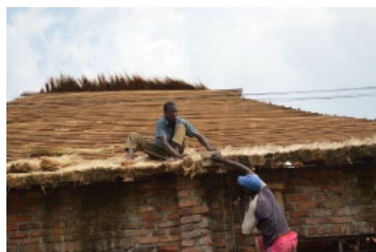
Thatch roof under construction in Sifukwe, Karonga. © Jon Twingi
