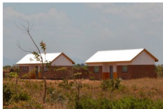
Houses with burnt brick walls, Reinforced Concrete beams and window sills, CGI sheets roof in Chisusu, Ntimba. © Jon Twingi
